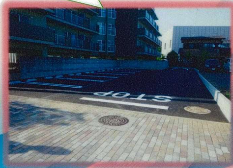
after (施工完了)
